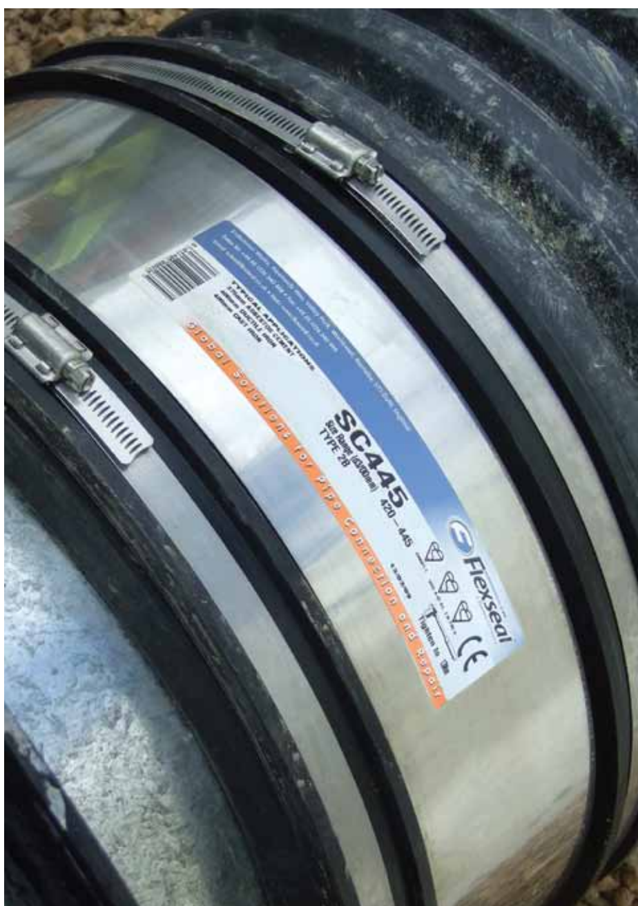
Connection of a 435mm Twinwall pipe into a 390mm stormwater tank using an SC445 and a BC24/390 bush
