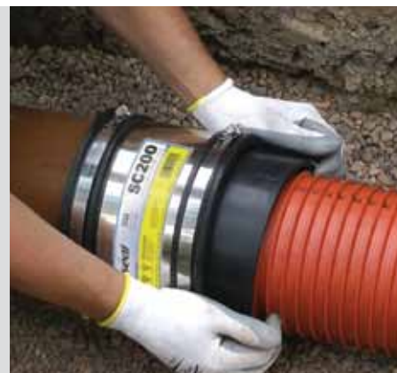
Connection of a 150mm clay pipe to a 150mm ultrarib using a BC08/170 bush
