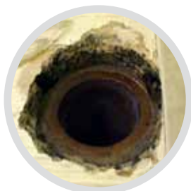
When a pipe is sheared close to a surface, with no stub or spigot
